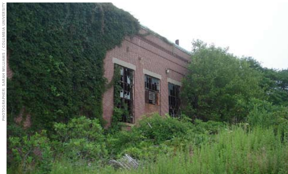
4.2.03 STRUCTURE AT FLOYD BENNETT FIELD, 2006
